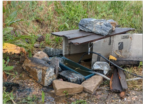
Figure 12. Plastic trough with stainless steel strainer installed in the eye bolts.
