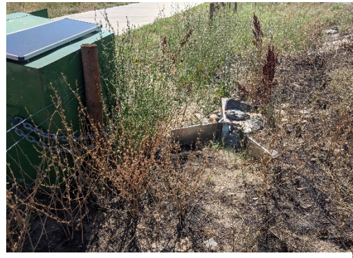
Figure 24. Vegetation at the ditch, burned after a small brush fire.
